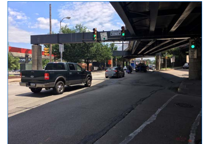
View of the intersection at East Carson Street, Arlington Avenue, and East Station Square Drive
