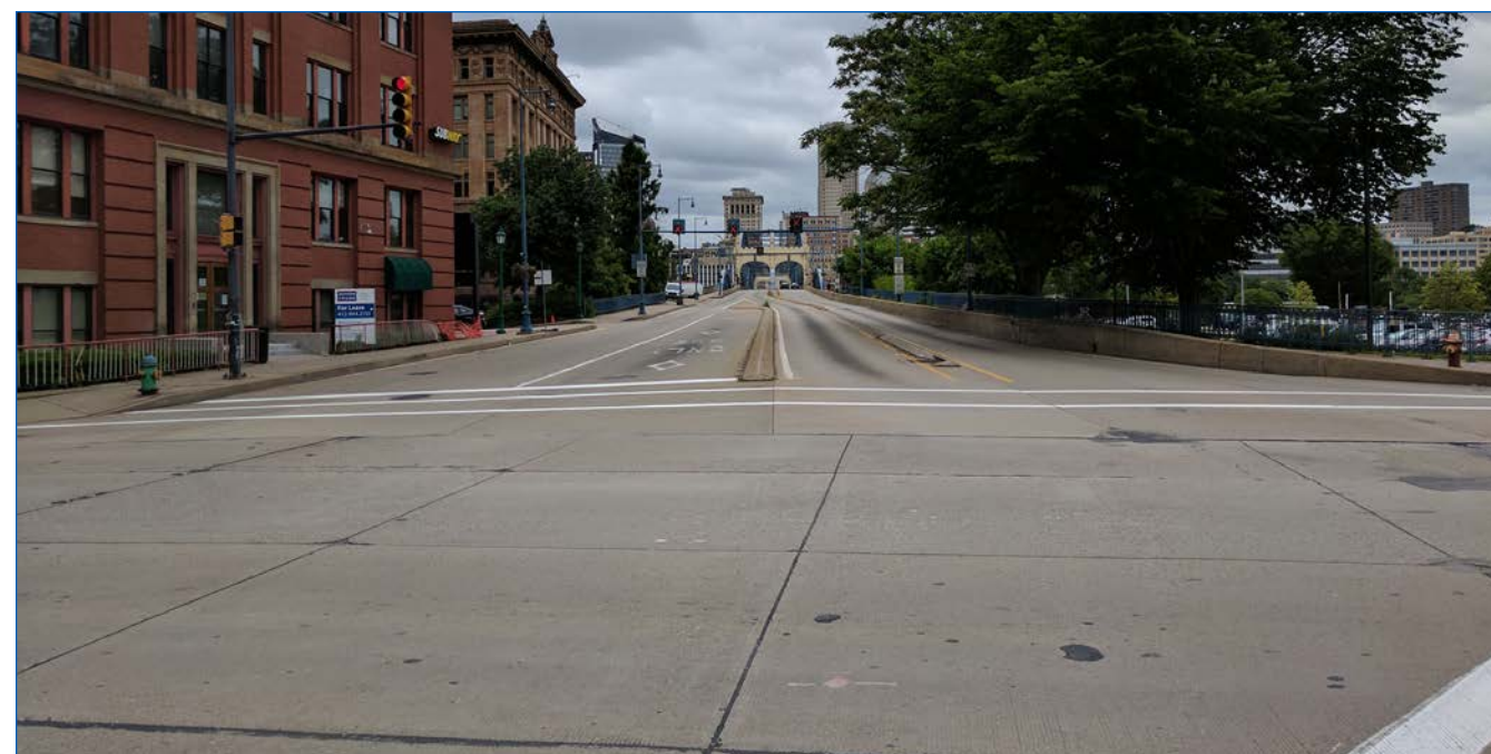
Intersection of Carson Street and Smithfield Street Bridge
