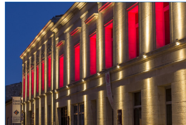
Lighting fixtures can be integrated within the landscape or carefully integrated with the facade. Small fixtures like these are barely noticeable from a distance. Source: platek.eu
