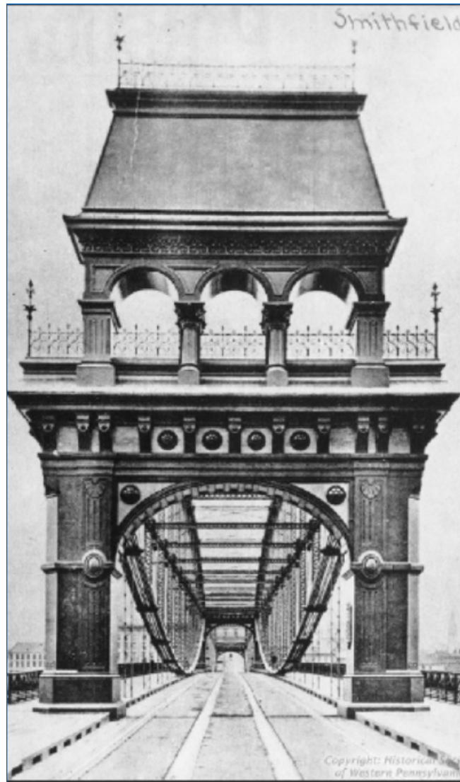
An early photograph of the Smithfield Street Bridge showing an entry portal before it was widened in 1911. Source: Jones and Laughlin Steel Corporation Photographs, Historical Society of Western Pennsylvania
