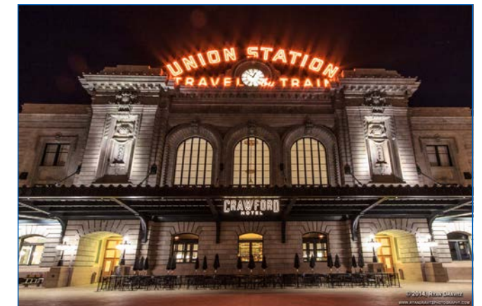
Modern architectural lighting was used in concert with historical fixtures and historic illuminated signage in the restoration of Denver's Union Station. Source: Urban Land Institute
