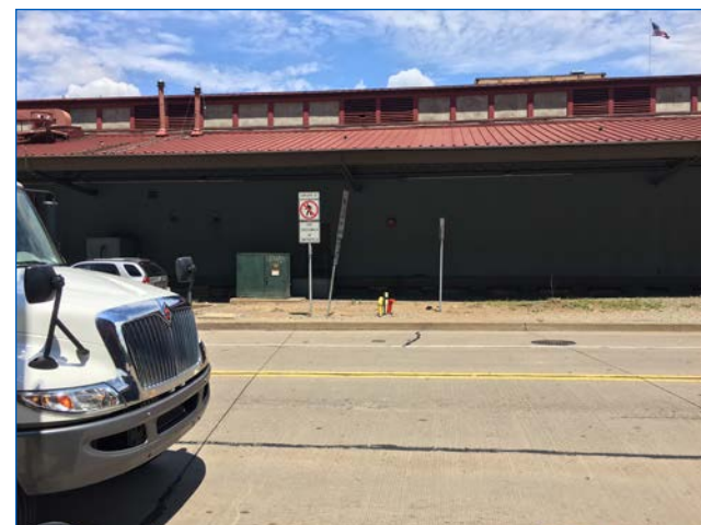
View upon exiting the Monongahela Incline Lower Station
