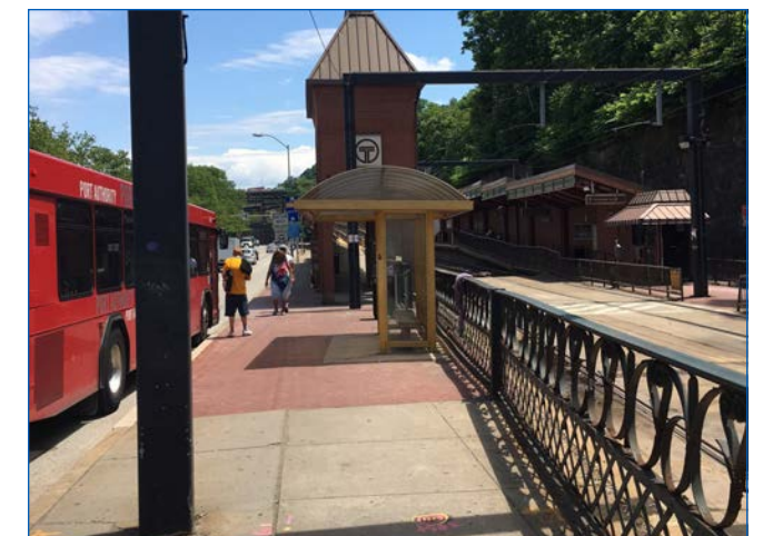
Looking east along East Carson Street at Station Square Station entrance
