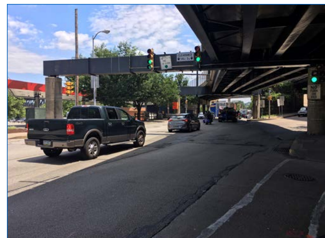
Arlington Avenue, East Carson Street, Station Square Drive, and the exit for the busway from the Transit Tunnel converge at one intersection
