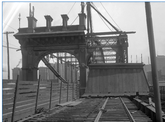
The top of the entry portals were removed in 1911 when the bridge was widened. Source: Pittsburgh City Photographer Collection, University of Pittsburgh
