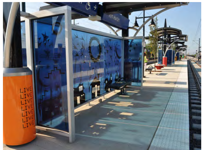
Side, perpendicular screens can help provide more protection, along with integrated artwork that provides extra shading and context. Tom Hunter Station, Charlotte
