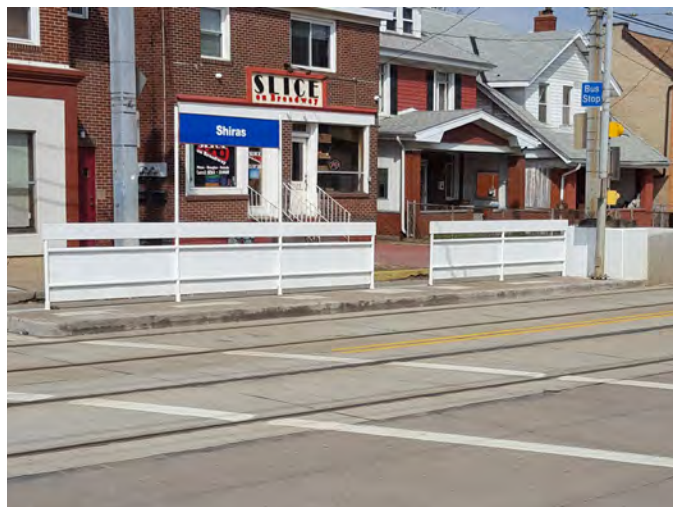
For stations with no canopy or overhead structure, mount Station Identification Signage on a vertical post, such as a light pole or provide one.
