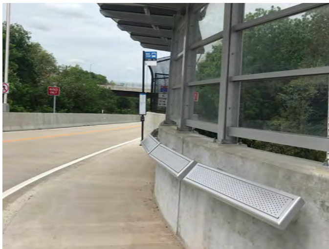
Covered leaning bar product along narrow boarding platforms should be mounted directly to the canopy structure. Neville Ramp Station, Pittsburgh
