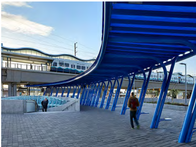
A covered walkway leads riders between the parking structure and the station platform at the Angle Lake Station, Seattle.
