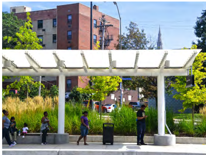
New canopy at East Liberty Station, Pittsburgh
