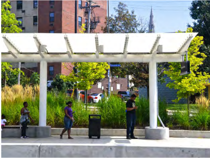
Station canopy at East Liberty Station, Pittsburgh
