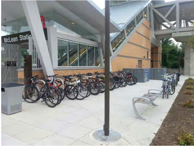
Utilize a mix of long- & short-term bicycle parking options, especially at suburban stations for downtown workforce commuters. McLean Station, Washington DC
