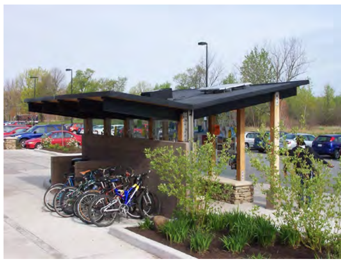
Utilize adjacent rooftop structures and disconnected downspouts for rainwater irrigation. Perkins Green Student Housing Complex bus shelter, Rochester
