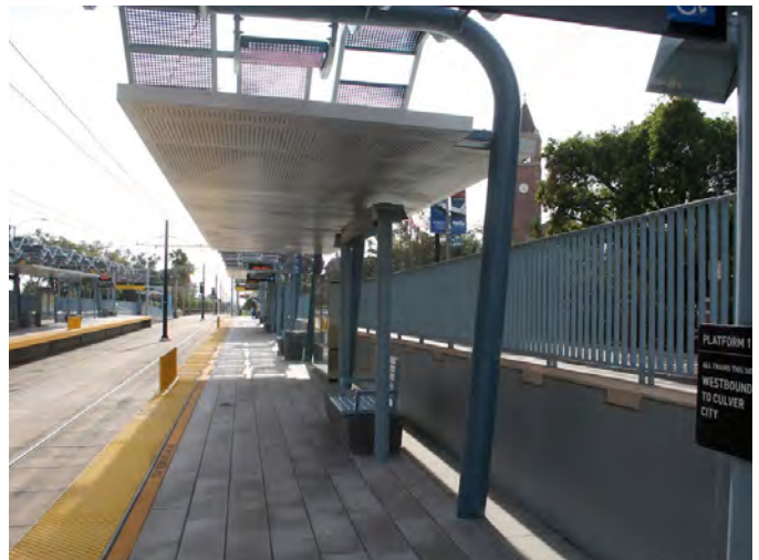
Common elements at Expo Park Station, Los Angeles
