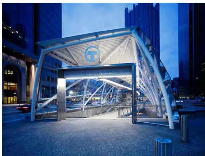
New entry & lighting at Gateway Station, Pittsburgh
