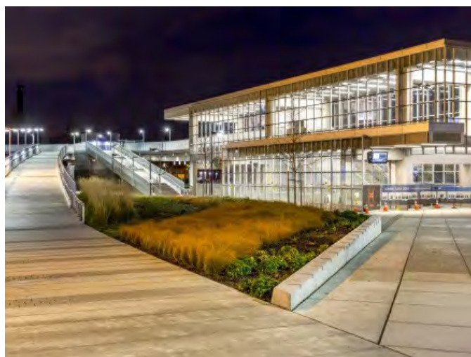
Site lighting at University of Washington Station, Seattle
