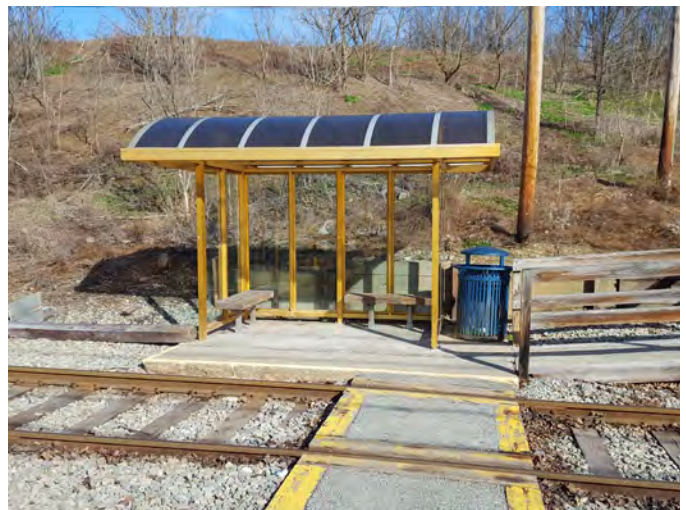
The LRT system contains highly diverse station facilities. Top: Gateway Station Middle: Dormont Junction Bottom: West Library Station
