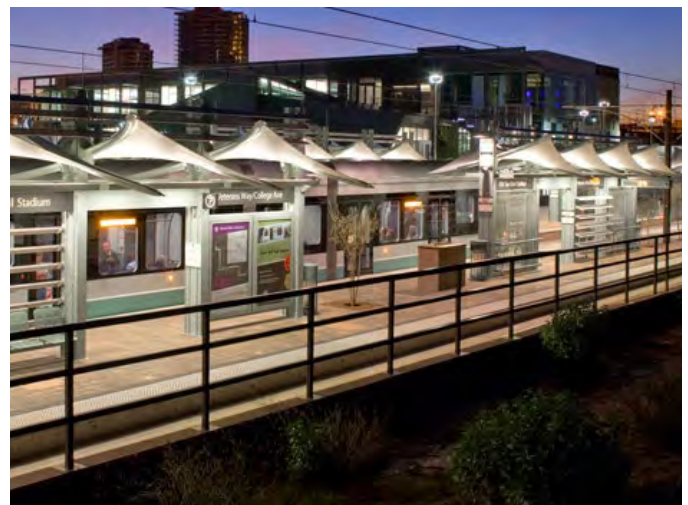
Platform and site lighting at Veterans Way/College Ave. Station, Phoenix
