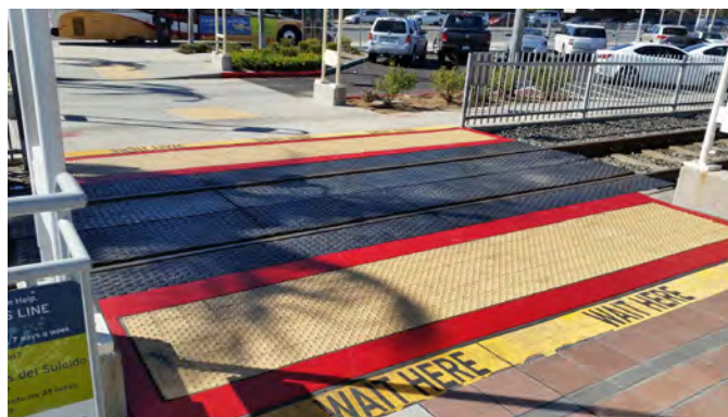
Use textured warning pavers and red paint to define the pedestrian track crossing. Wardlow Station, Los Angeles
