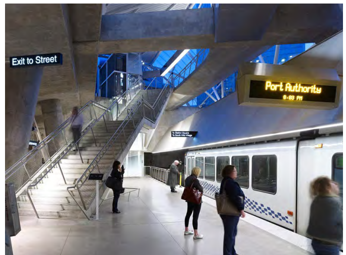
Tough materials and protective coatings at Gateway Station, Pittsburgh
