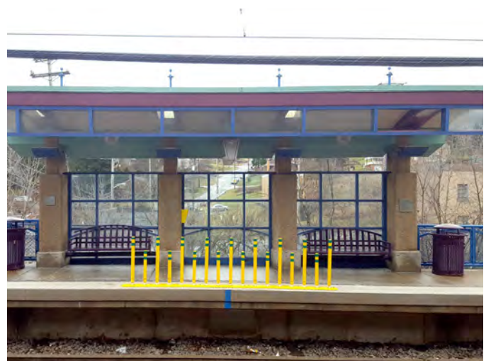
Existing standard between car barrier at McNeilly Station, Pittsburgh
