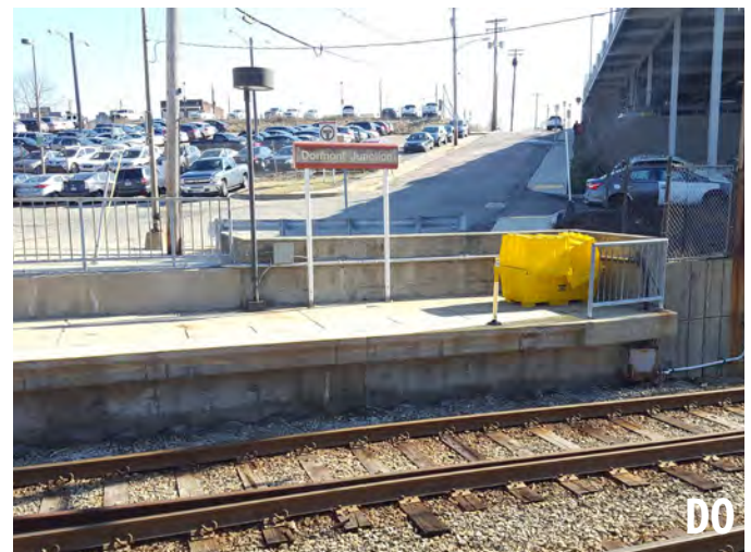
Existing mid-platform salt storage bin at Dormont Station is placed at the end of the platform, out of the way of pedestrian accessibility and clear of sight lines.
