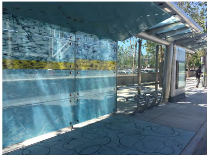
Incorporate design into windscreens and paving. Merge Conceptual Design's Room Within windscreen and pavement at Arena BRT Station, San Jose
