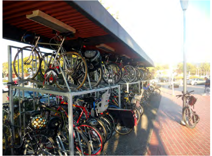
For short-term parking, consider covered, structured exterior bicycle parking to increase capacity with limited space. North Berkeley Station, Berkeley
