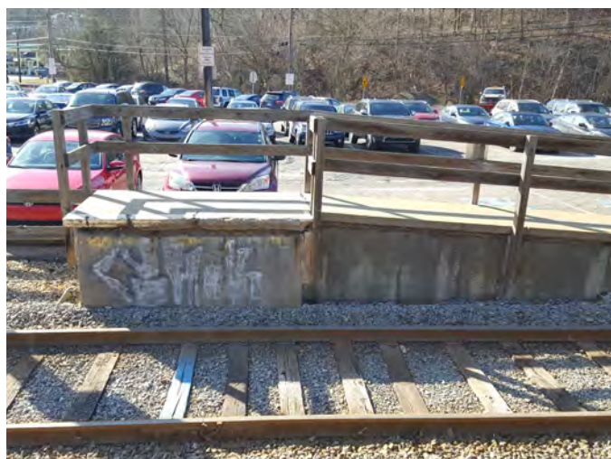
West Library Station
