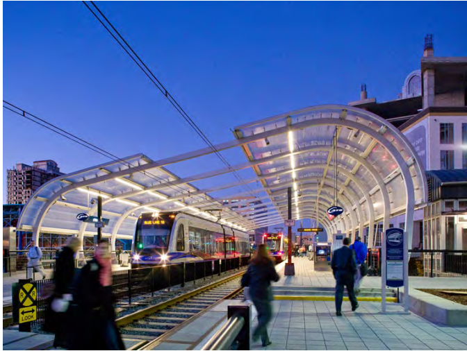
Stations with limited property can utilize platform adjacent entry plazas to directly connect public right-of-ways with the platform. CTC Station, Charlotte
