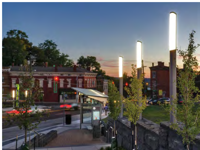
Site lighting should also visually help lead users along primary paths by creating a line of light. Lower bollards or step lights are more focused and directional.
