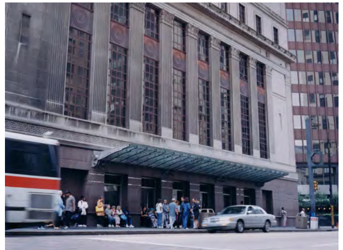
Station adjacent bus stops should feature a shelter or canopy that relates to the light rail station design & architecture. Wood Street Station, Pittsburgh
