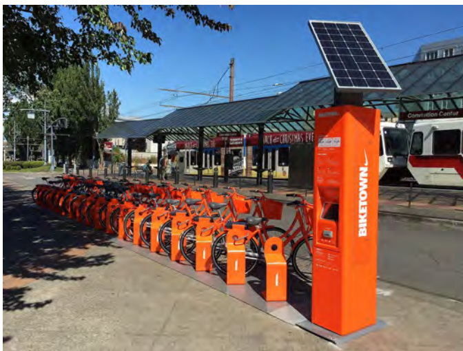
Consider each bike-share system's installation needs, such as solar power or required installation clearances. Biketown bike-share station at Convention Center MAX Station, Portland
