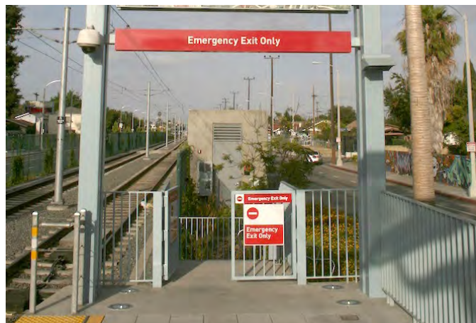
Use signage and color directly on end access and emergency exit gates. Expo/Western Station, Los Angeles
