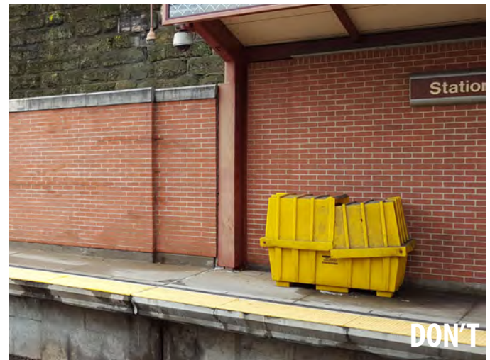
Existing mid-platform salt storage bin at Station Square limits accessibility, blocks sight lines, and attracts debris accumulation.
