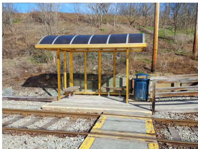
West Library Station
