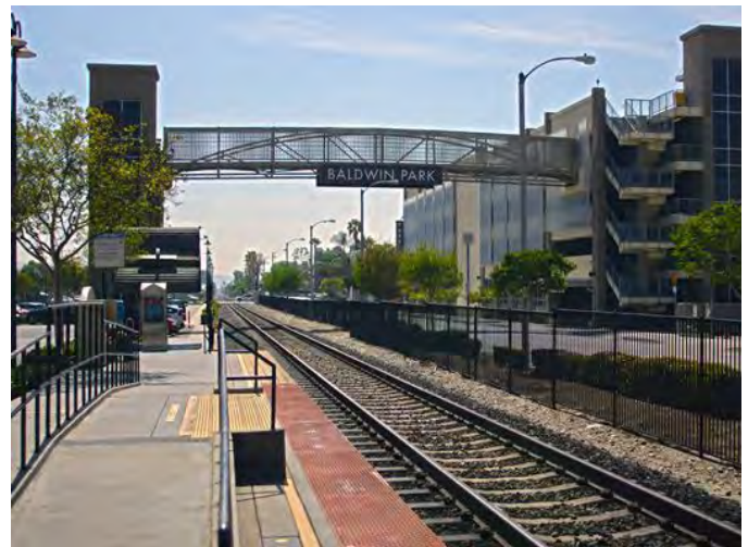
For high-investment, high-volume stations with parking structures, consider connections which reduce pedestrian safety issues. Parking garage and platform connection at Baldwin Park Station, Los Angeles
