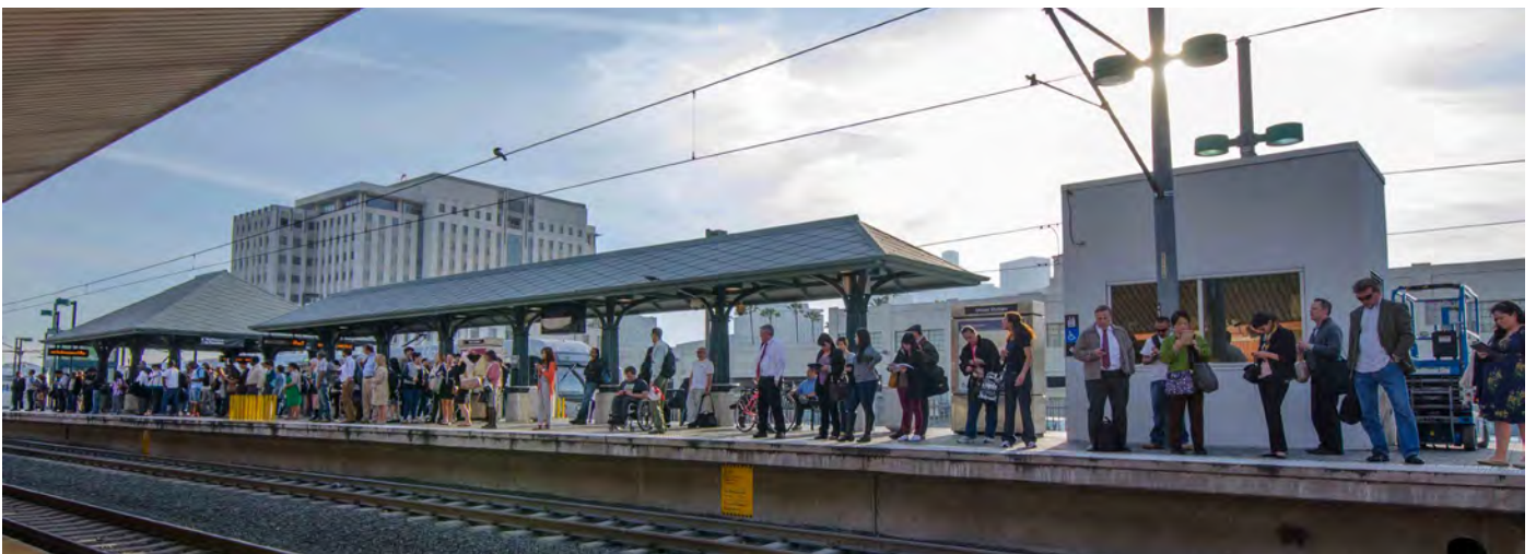
Central, traffic separated platform at Union Station, Los Angeles
