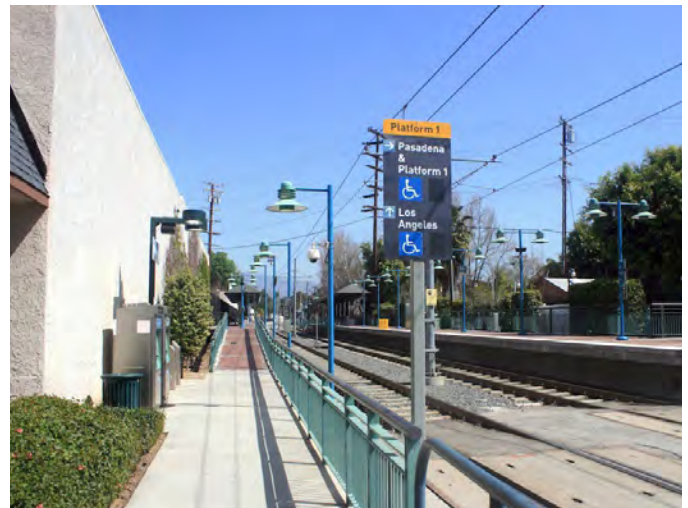
ADA Signage should be placed along the station property to direct arriving riders the accessible routes to the platform. South Pasadena Station, Los Angeles
