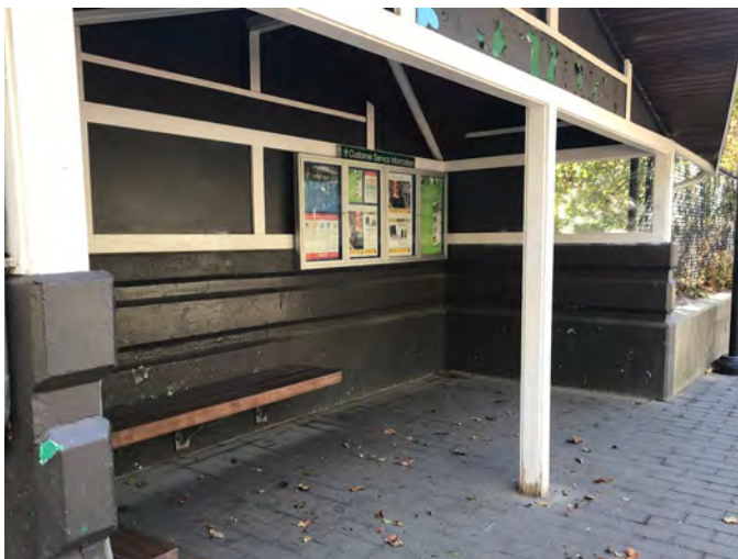
Patron Notice Board under covered platform shelter at Longwood Station, Boston
