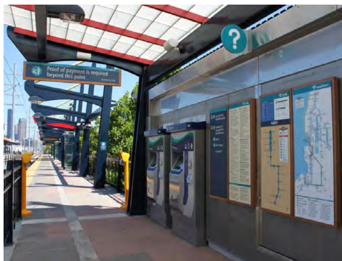
Information kiosks which includes ticket kiosks, maps, schedules, and notices. Sodo Station, Seattle
