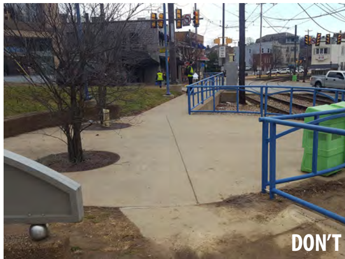
Existing entry plaza at Willow Station, Pittsburgh is narrow, constricted, and cluttered.
