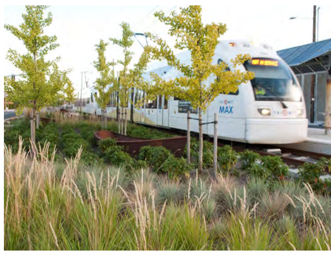
In place of safety fencing, couple planting and public art, such as sculptures, to act as barriers and safety separation. SE 17th Ave & Rhine St. Station, Portland
