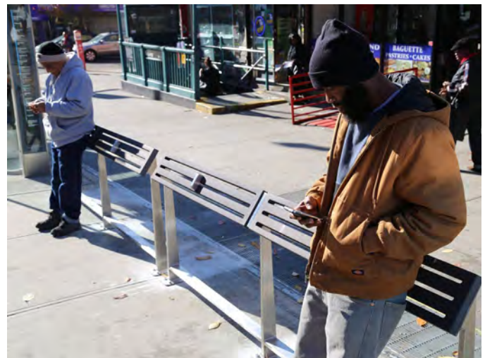
Along narrow platforms or high-volume stations, provide freestanding leaning bars in place of benches to save space. Nostrand Ave. bus stop, New York City
