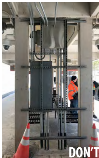
Left: Conduit and electrical boxes clutter the platform at Mt. Lebanon Station. Right: Electrical and data wires are integrated into structures at North Side Station.
