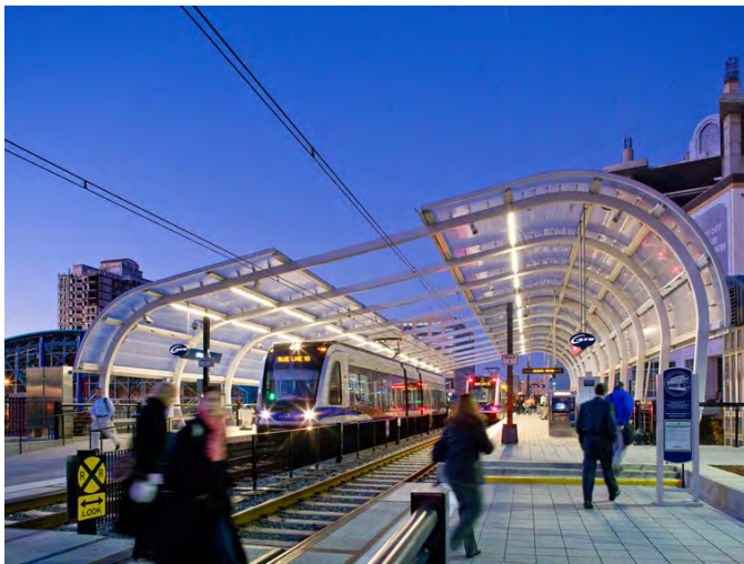
Station entry plaza, Charlotte
