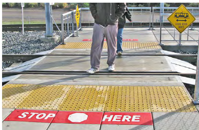
Consider incorporating upright signage, in addition to text on the ground, to define track crossing and ramps. Lents / SE Foster Rd Station, Portland
