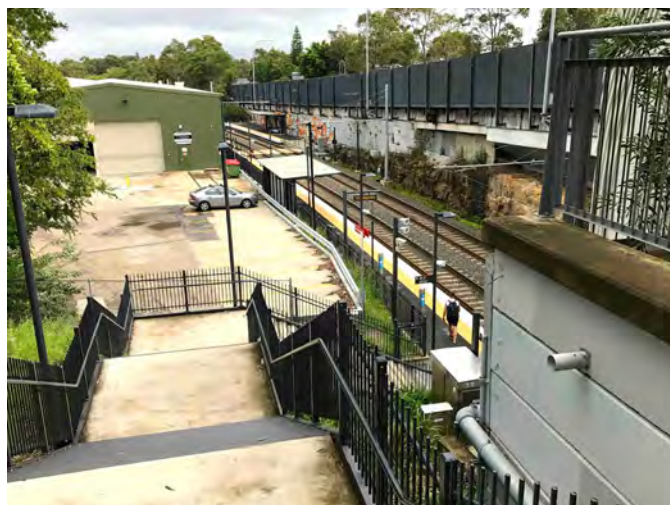
Direct platform access with integrated elevator at Leichhardt Station, Sydney
