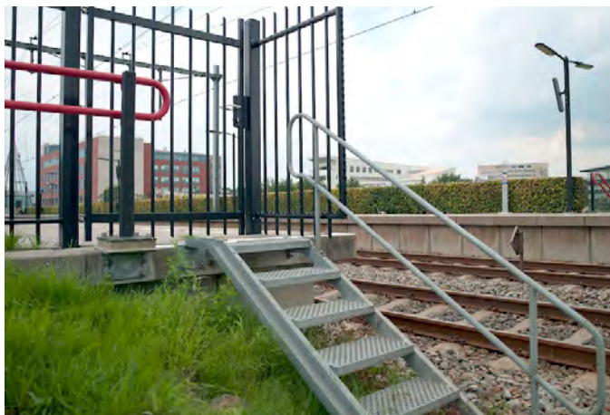
To not interfere with passing trains, end platform fencing should terminate a safe distance away from the platform edge and utilize a perpendicular section to deter riders from passing around. Netherlands
