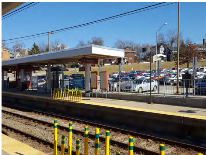
Existing elevated, long Dormont Junction platform and canopy
