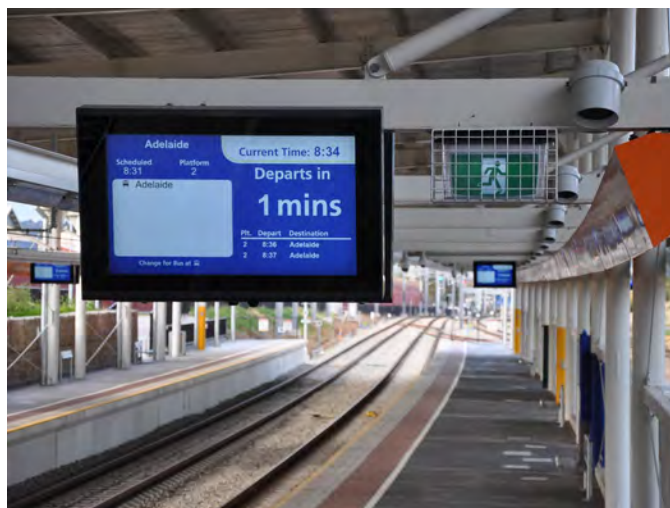
For high investment stations, Real-Time Arrival Information displays shall be vertically-mounted, parallel to the tracks, near waiting areas. Adelaide, Australia
