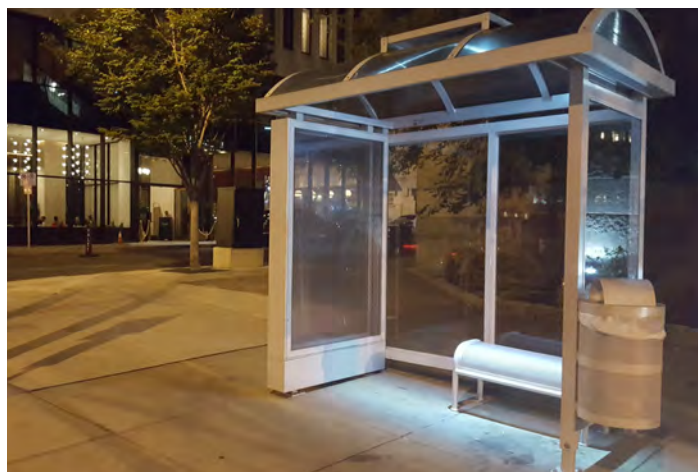
Lighting at a Shelter Stop in Nashville
