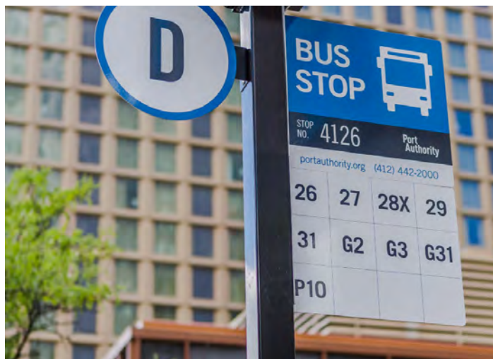
New Style PAAC Bus Stop Sign in Process of Being Installed
