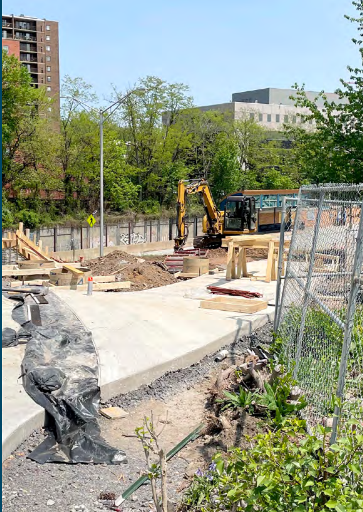
Negley Station under construction (Spring of 2022)
